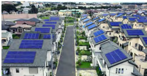
Sharp solar power systems on homes in a housing development in Chiba Prefecture, Japan
