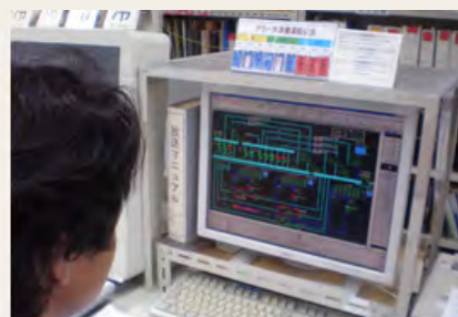
Checking the operational status of air-conditioning units
